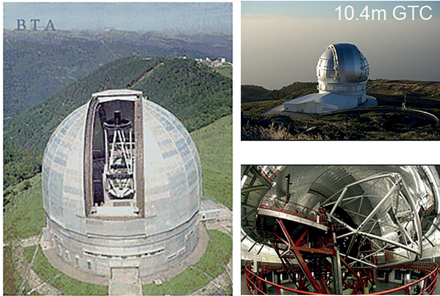
Fig 7. Left: The dome of the 6-meter BTA telescope of SAO RAS. Right: The dome of the 10.4-meter Gran Canarias Telescope (GTC) (top) and the telescope itself (bottom).
